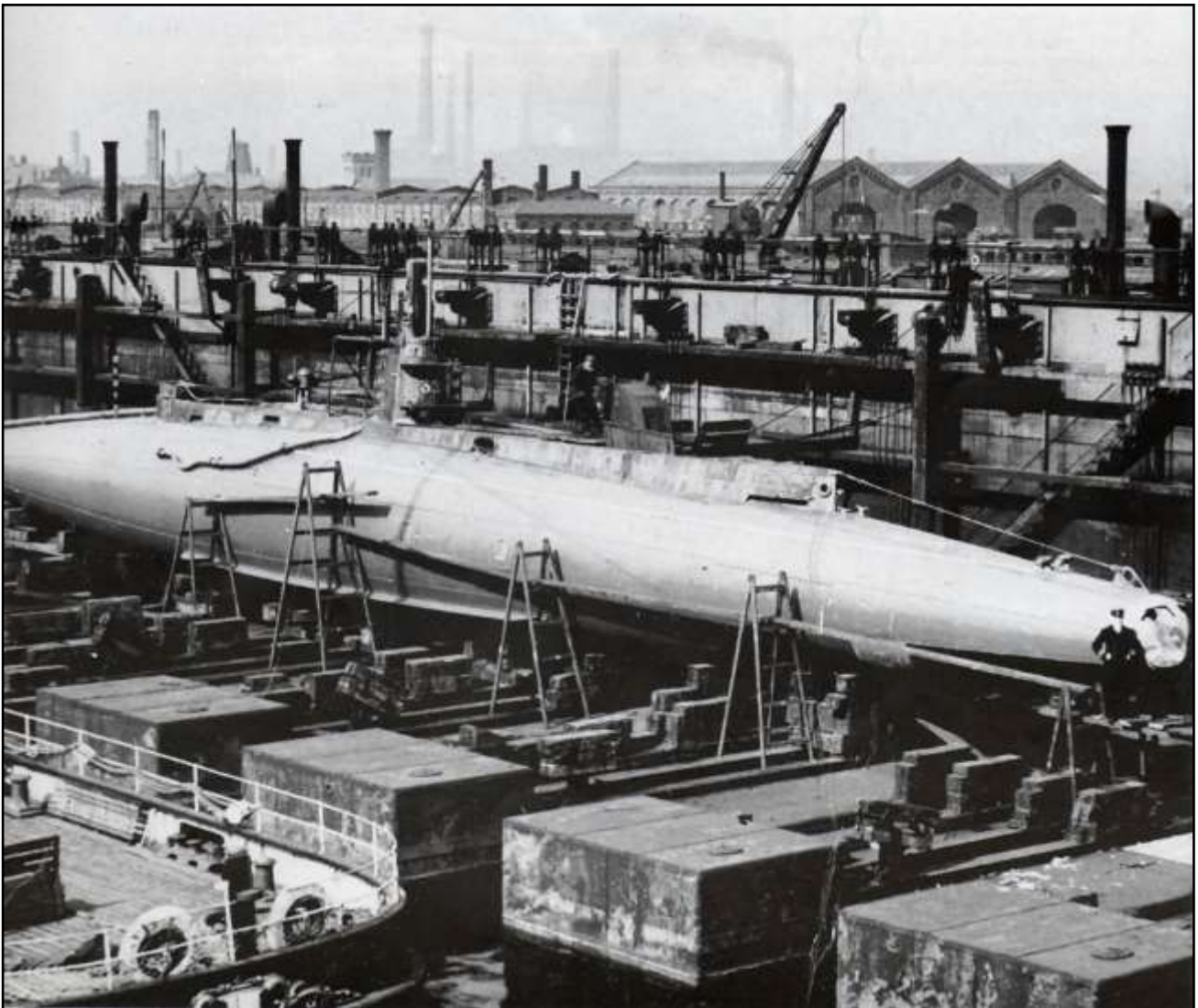
B Class submarine being fitted out in Devonshire Dock.
