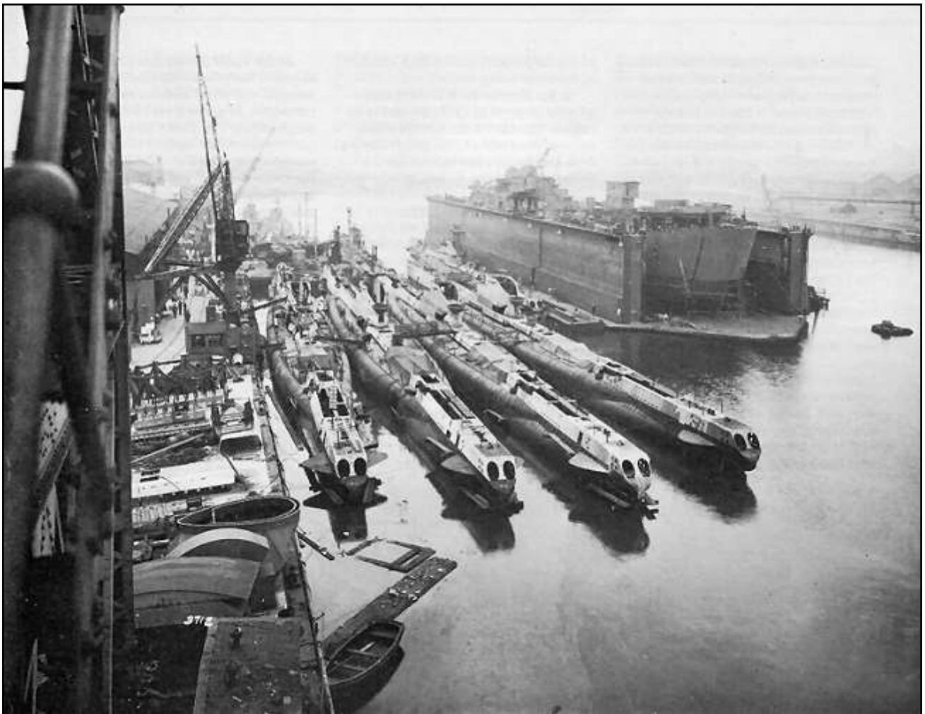
A Class submarines at various stages of fitting out.
